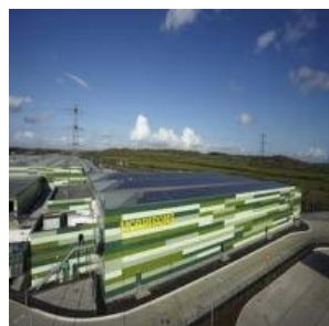
Morrisons Distribution Center (UK)
